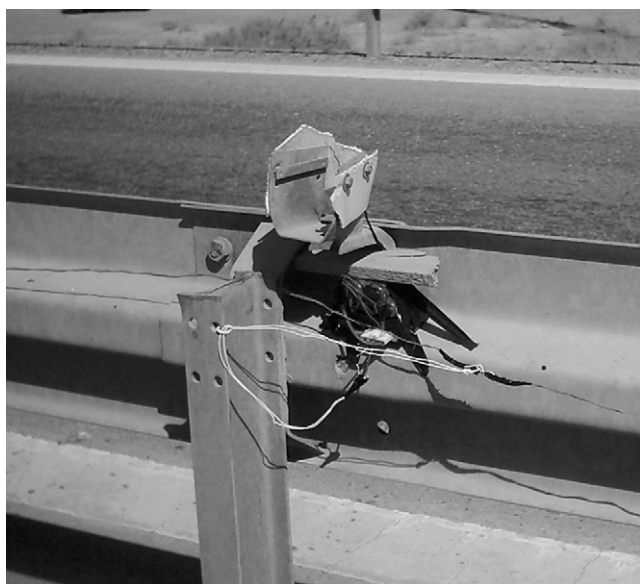
FIGURE 65-1. Garage door opener detonation device (notice wire).
